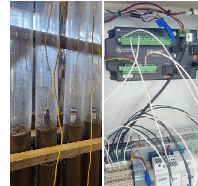
TDR Water sensors and CR6 data logger to record soil VWC%
